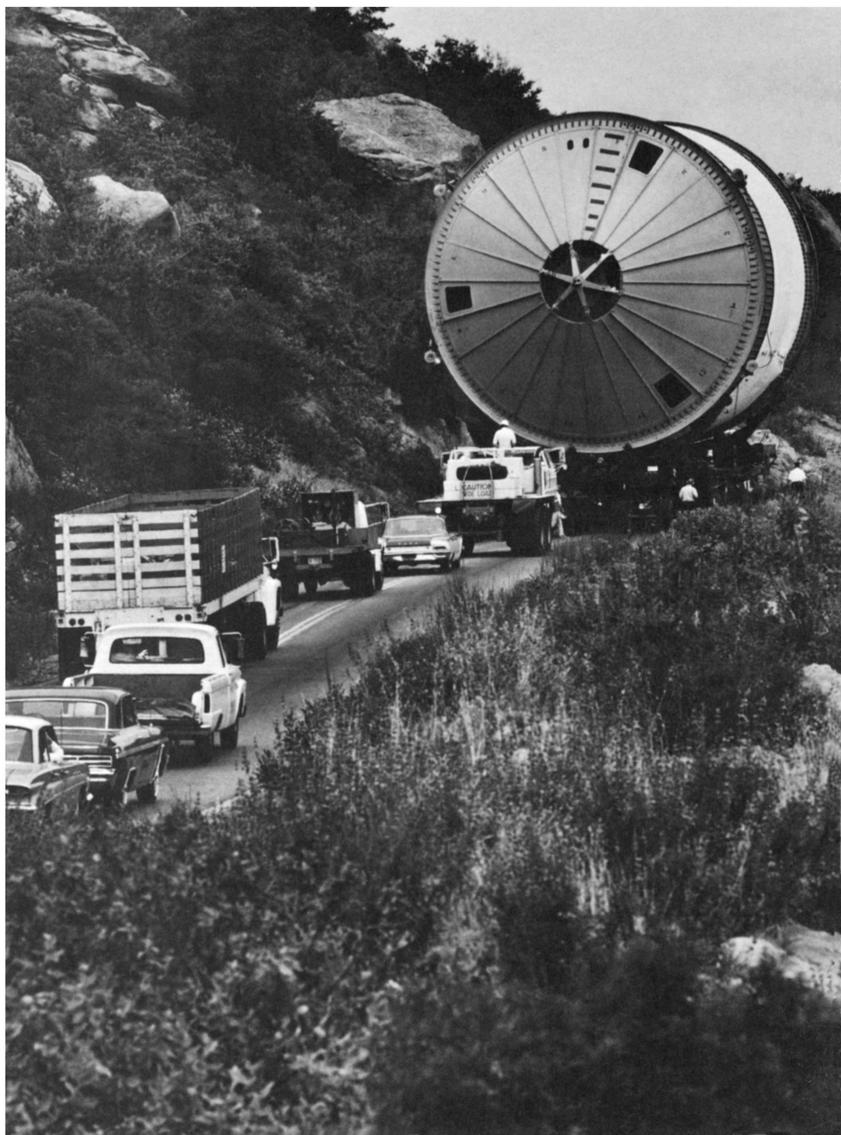
Top left, the common bulkhead test tank is 47 feet long, 33 feet in diameter. The complete Saturn S-II, being built by Space Division for NASA is 81½ feet long. Four concentric rings in base are specially installed for pressure test data.
