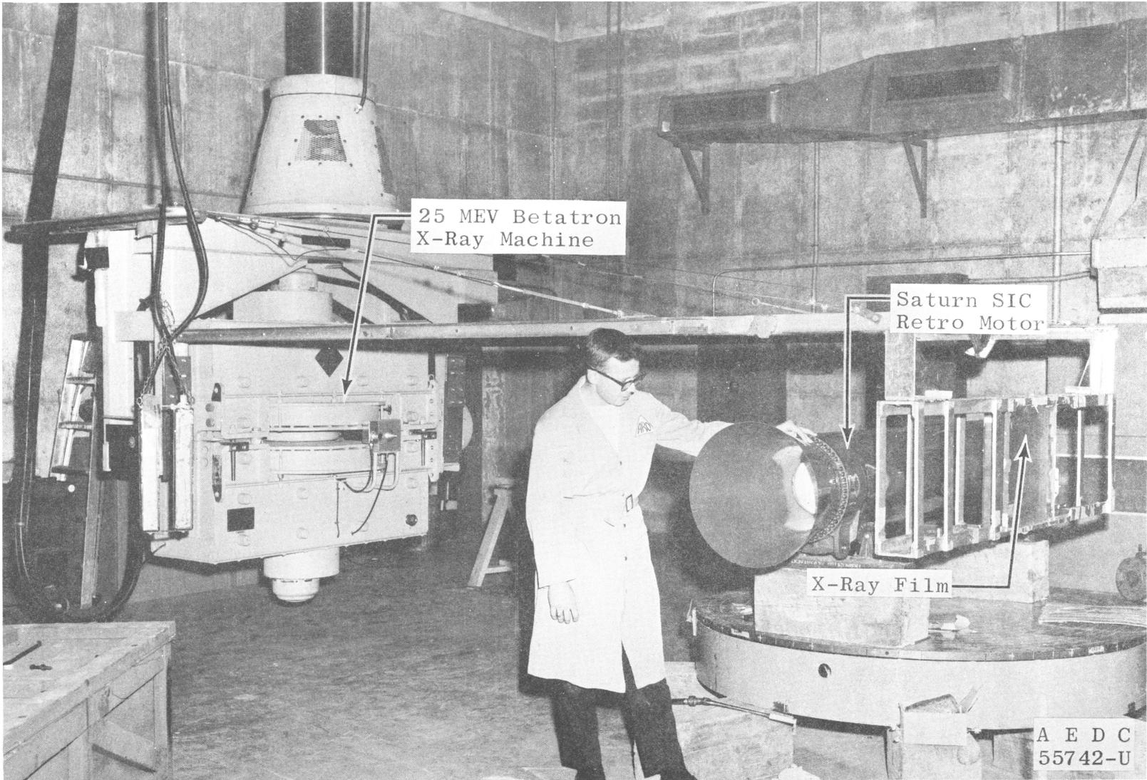
Fig. 5 Saturn SIC Retro in X-Ray Inspection
