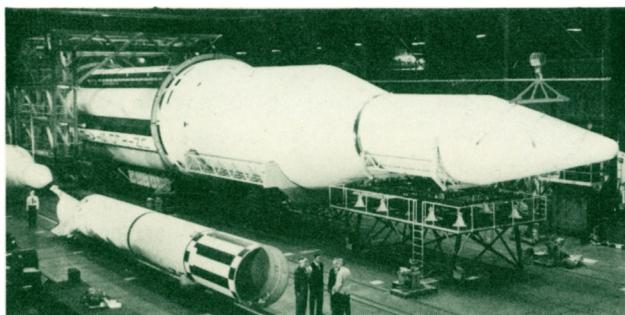
Marshall's current projects include the following space vehicles and stages: Saturn C-1, Saturn C-1B, Saturn C-5, Nova, Thor Agena-B, Atlas Agena-B, and RIFT (Reactor-in-Flight-Test). The engine development projects which Marshall is directing include the H-1 and F-1 engines, using the conventional liquid oxygen and kerosene fuel combination, and the RL-10 and J-2 engines, which use the high energy propellant combination, liquid hydrogen and liquid oxygen.
