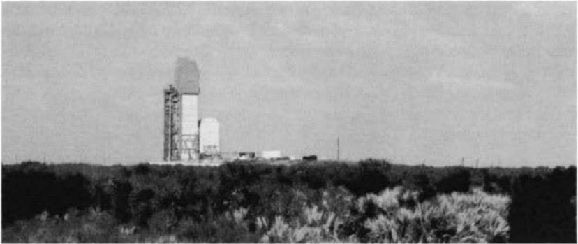
On RIGHT, Complex 19, while similar to 15 and 16, has been greatly modified in preparation for the Gemini two-man space capsule program. The solid "red-room" at the top of the larger erector is the controlled environment enclosure for the Gemini capsule. Titan II will serve as the booster in this program just as did Atlas in the old Project Mercury.
