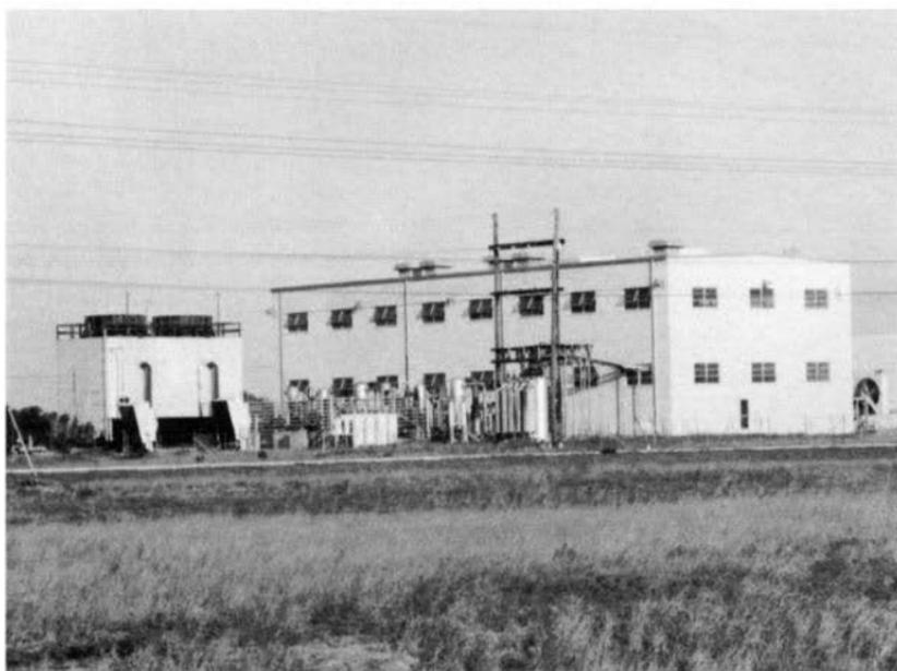
On LEFT you will see a two-story gray building with large outside plumbing. This is our liquid-oxygen-producing plant. Liquid oxygen, or LOX as it is commonly called, is the oxydizing agent used in combination with highly-refined kerosene to fuel such missiles as the Atlas and the Thor. The convenient on-Cape location saves transporting the very cold (-297.9 degrees Fahrenheit) LOX over public highways.
