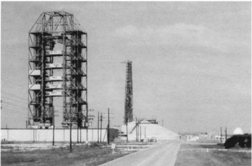
On RIGHT, as you turn left onto Cape Road, stand the two largest known movable structures in the world, the Saturn gantries on Complexes 34 and 37. The nearer tower of Complex 34 stands 310 feet tall, or as tall as a 31-story building. The structure at Complex 37 stands six stories taller at 375 feet. The huge Saturn will play a key role in the lunar landing program of the National Aeronautics and Space Administration (NASA).
