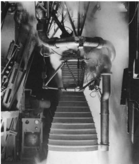
H-1 Engine Test Firing
