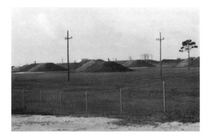
TO YOUR RIGHT are stored the various stages of solid propellant missiles, which must be treated as high explosives. The square concrete building to the rear, which may be flashing a red light, houses one of the world's largest x-rays, used to seek out possible flaws in the missile's solid propellant.
