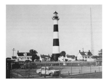
On IEFT, and very prominent, is the 165-foot black and white striped lighthouse. This lighthouse has been a Cape landmark since it was built in 1868. Constructed originally of wood, it was later rebuilt with riveted steel plates lined with brick. From a distance this structure greatly resembles a missile and more than one hapless newcomer to the Cape - invited to watch a missile launch - has kept his eyes glued to the lighthouse while the real missile lifted off from an entirely different area.
